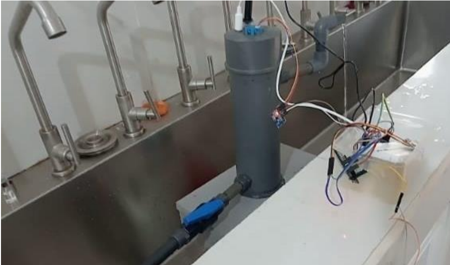
Figure 3.1: Real-time Monitoring at Water Treatment Plant Inlet
